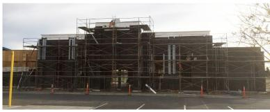
The Pierce High School's new multi-purpose building continues to take shape with the exterior lath & plaster materials being installed. On the interior of the building, major components for electrical, fire sprinkler and plumbing are being installed. On February 15, 2018, approximately 25 students toured the new multi-purpose building and were invited to be part of interior space planning process. The students were given opportunities to ask questions about the construc-
